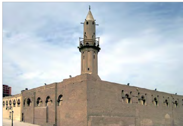
ʿAmr ibn al-ʿĀṣ Mosque, Egypt's oldest mosque, Cairo Flickr/David Stanley
