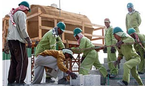
© Richard Messenger Construction workers
