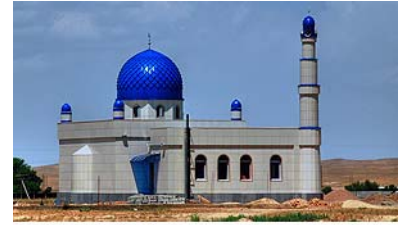
© Irene2005 / flickr.com Mosque construction
