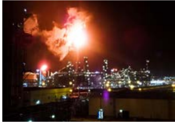
V Chemical plant in Skikda Flickr / Stefano F
