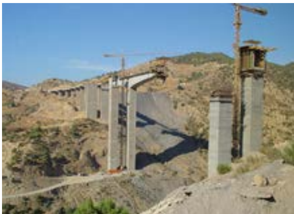
New bridge construction near Ain Turk. Public Domain
