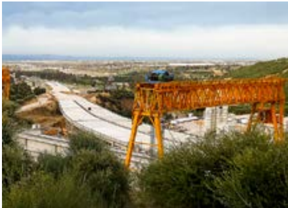
Road construction Sidi Madani Public Domain
