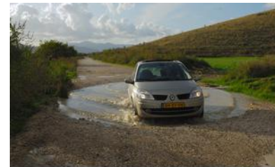
© Rob Hogeslag Rural roads in poor condition
