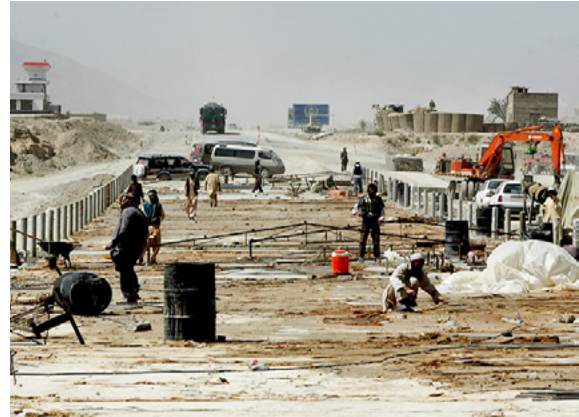
Building the Gardez-Khost road in Jadran, Paktia Province Flickr/USAID Afghanistan
