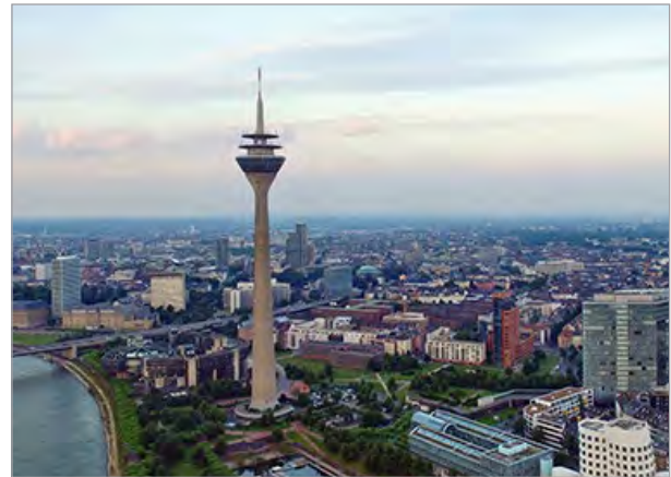
Rheinturm telecommunications tower, Düsseldorf Pixabay / nokidoc
