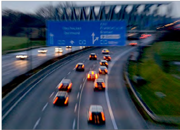
Autobahn A2 near Dortmund Flickr / Dirk Vorderstrasse
