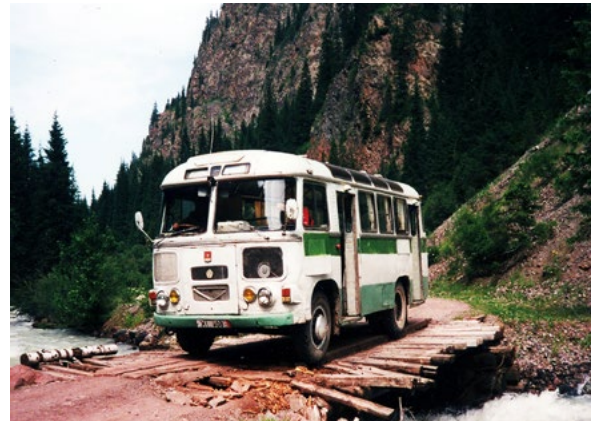
Bus attempting to cross a narrow bridge Flickr / shirtpants
