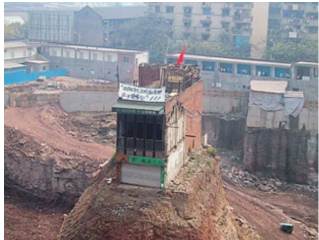
A nail house, whose owners refuse to leave, preventing construction of a shopping mall, Chongqing Wikimedia/zola
