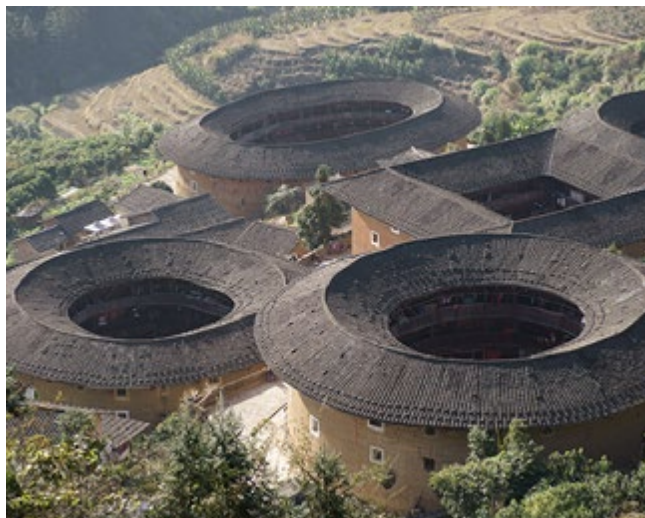
Tianluokeng cluster of circular and rectangular tulou, UNESCO World Heritage Site, Zhangzhou City, Fujian Province Flickr/notch
