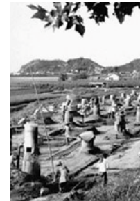
Courtesy of Wikipedia.org Backyard furnaces
